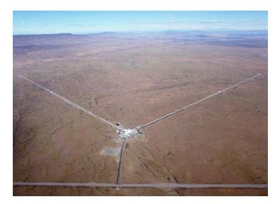
LIGO's antennas are L-shaped, with perpendicular arms 2.5 miles long. Inside each arm, cocooned in layers of steel and concrete, is a vacuum chamber two feet wide containing 2.5 million gallons of empty space. At the end of each arm is a mirror hanging by glass threads.
